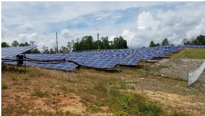
*Example of a fixed tilt installation in Conyers, GA on solid rock with ground screw foundations*
