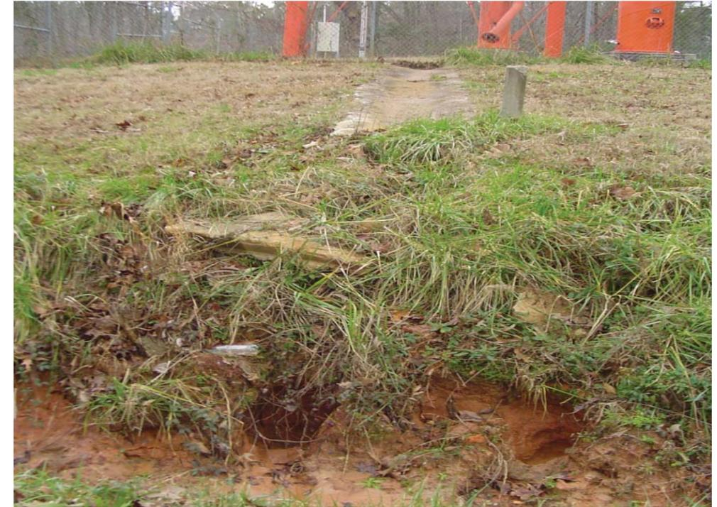
*Erosion from pipe draining water tower*
